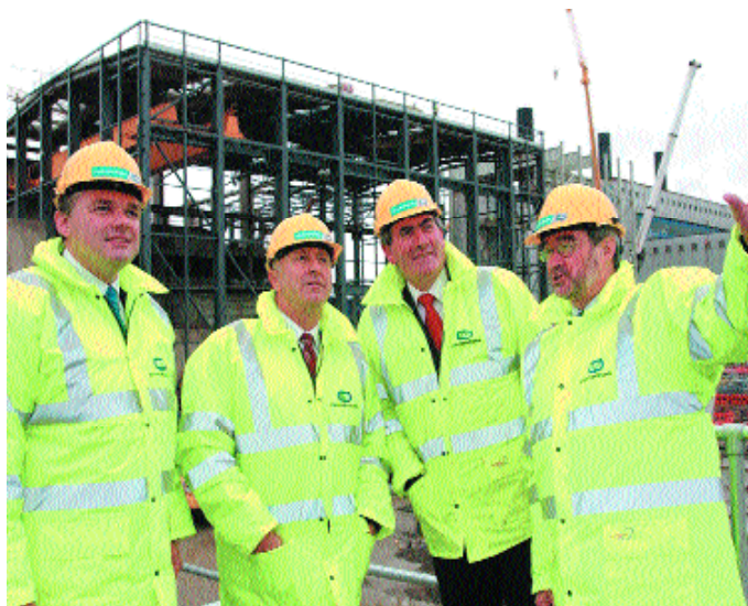
Minister Ian Pearson MP, Minister Dermot Ahern TD with Padraig McManus, ESB Chief Executive, and Richard Sterling, Managing Director CPL, on a visit to the site at Coolkeeragh ESB
