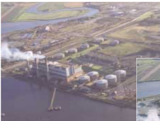
Existing oil fired station
